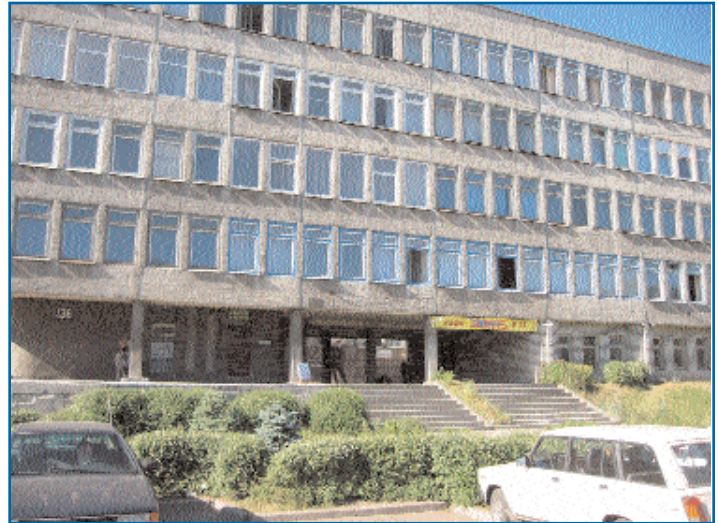
Building in the city of Kaliningrad housing Jarvis Skandinavien AB's new branch office that's serving all of Russia.
